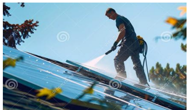
Fig 3. Water Based Cleaning
